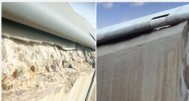
Precast Concrete panels with exposed reinforcement treated and repaired to original.
